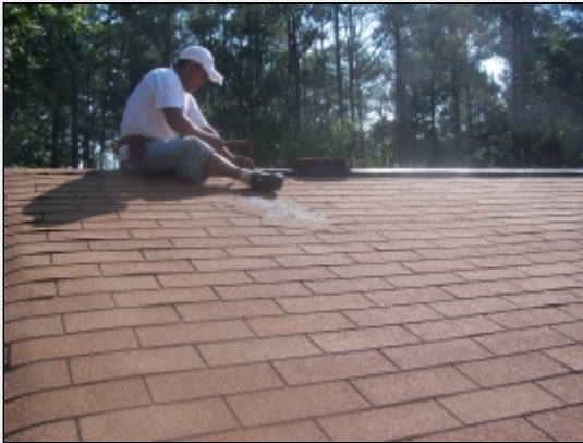
install new shingles over vent
